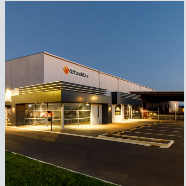
Christchurch distribution center
